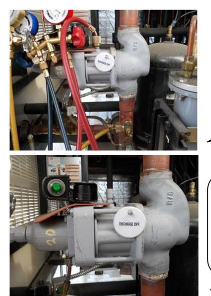
When setting the valve first <u>hook</u> up two high s<u>ide</u> gauges before and after the <u>valve</u>.
