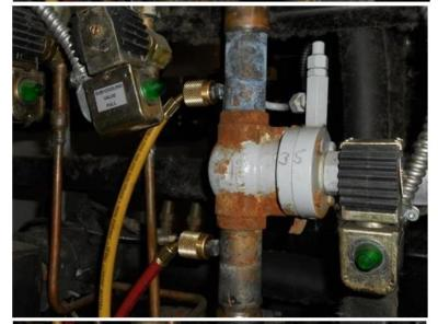
This is an example of an OLDR valve in a Super Target inside the PUC. The valve can be found on the liquid line after the sub-cooler.
