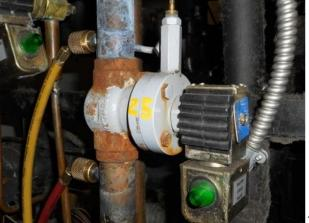
Adjust valve until Target's 20-25 <u>pound</u> differential <u>setting</u> is achieved. Watch gauges for 5 to 10 min to <u>ensure</u> valve is holding differential. After valve is <u>set</u> document on valve the pressure setting with a <u>paint</u> marker. Once you are completed make <u>sure</u> ball <u>or</u> king valve is opened for hot or cool gas line!!
