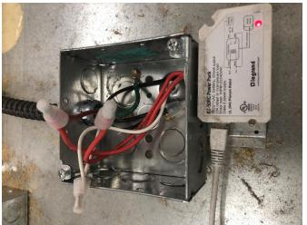
If case has motion detection below), remove jumper and override power pack as described above
